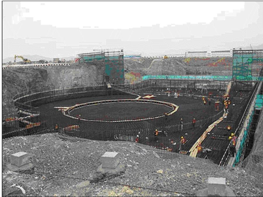
**Figure 3:** construction of the first AP1000 at Sanmen NPP site in China
