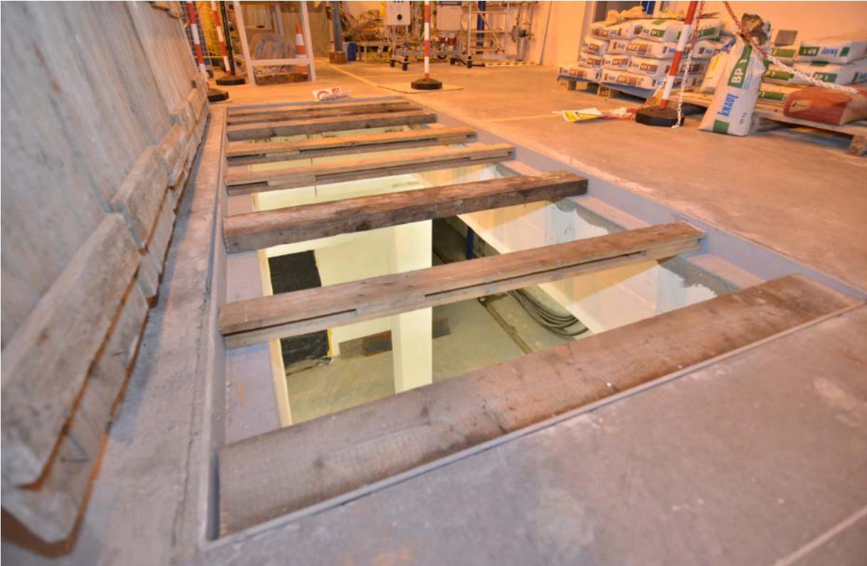
Fig. 9 Photo of rectangular floor opening for the cooling channel installation.
