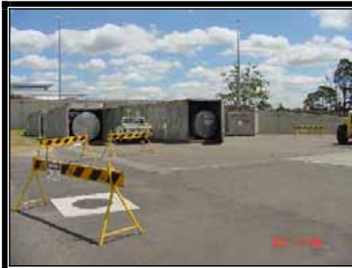
Cask Receipt/Inspection/Unloading Area
