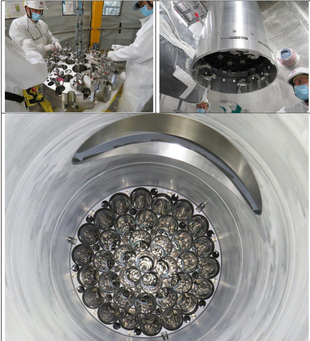
Figure 15: Jules Horowitz Reactor Block - Final setting of some internals
