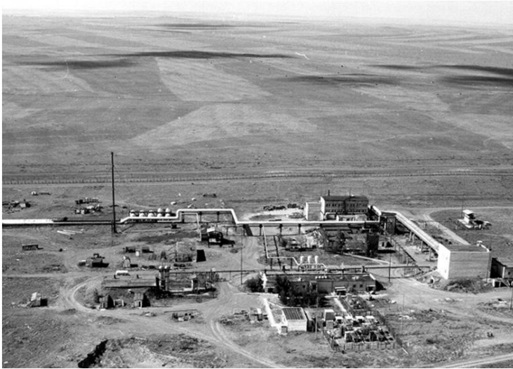
Figure 1. The IGR Reactor Complex
