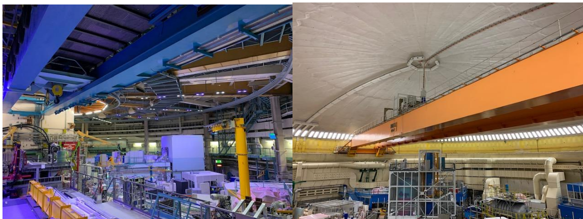
Fig 9. Overhead crane on Level C and polar crane on Level D
