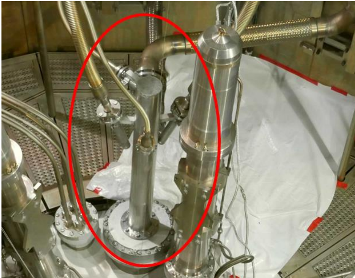
Figure 4: The dummy mounted at the place of the CNS (encircled in red). Prominent to the right is one of the shut-down rods, another one barely visible on the bottom left. The thicker flexible lines in the back were and will be used to supply vacuum and liquid deuterium. The medium one on the left is a helium supply line (the other one hidden behind the shut-down rod). The bellows in front hoses electric lines for instrumentation.
