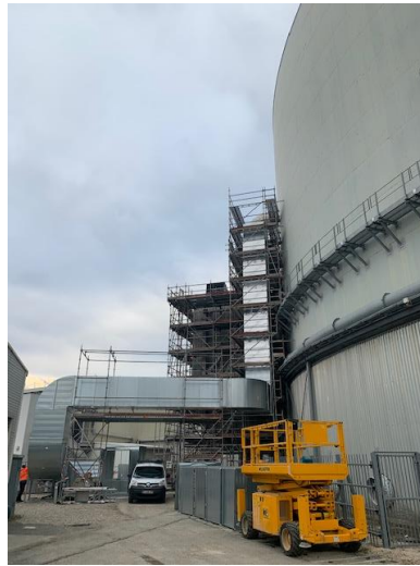
Fig 10. Rebuilding of the fresh-air intake
